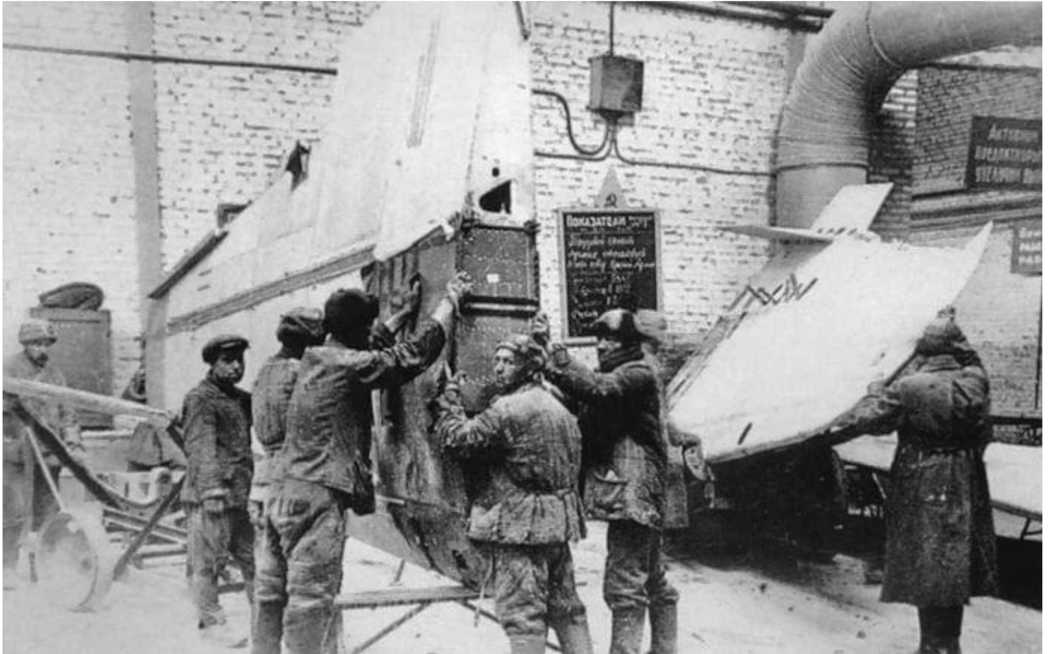
Series 2 – mixed (metal and wood) design of the wing console
